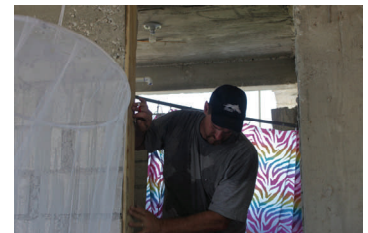
Jan Tonkin installing a door on one of the new bathrooms.
